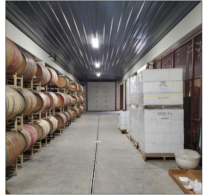
LIGHT BAR – WINERY STORAGE ROOM
