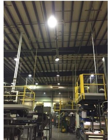
In one other production area with the need for very precise lighting, and also at a higher ceiling height (approximately 23 feet), the 200-watt Ice Breaker High Bay was utilized and again yielded exceptional output and approximately 30 foot-candles of light. 109 of these units were used.
