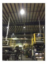
In one other production area with the need for very precise lighting, and also at a higher ceiling height (approximately 23 feet), the 200-watt Ice Breaker High Bay was utilized and again yielded exceptional output and approximately 30 foot-candles of light. 109 of these units were used.
